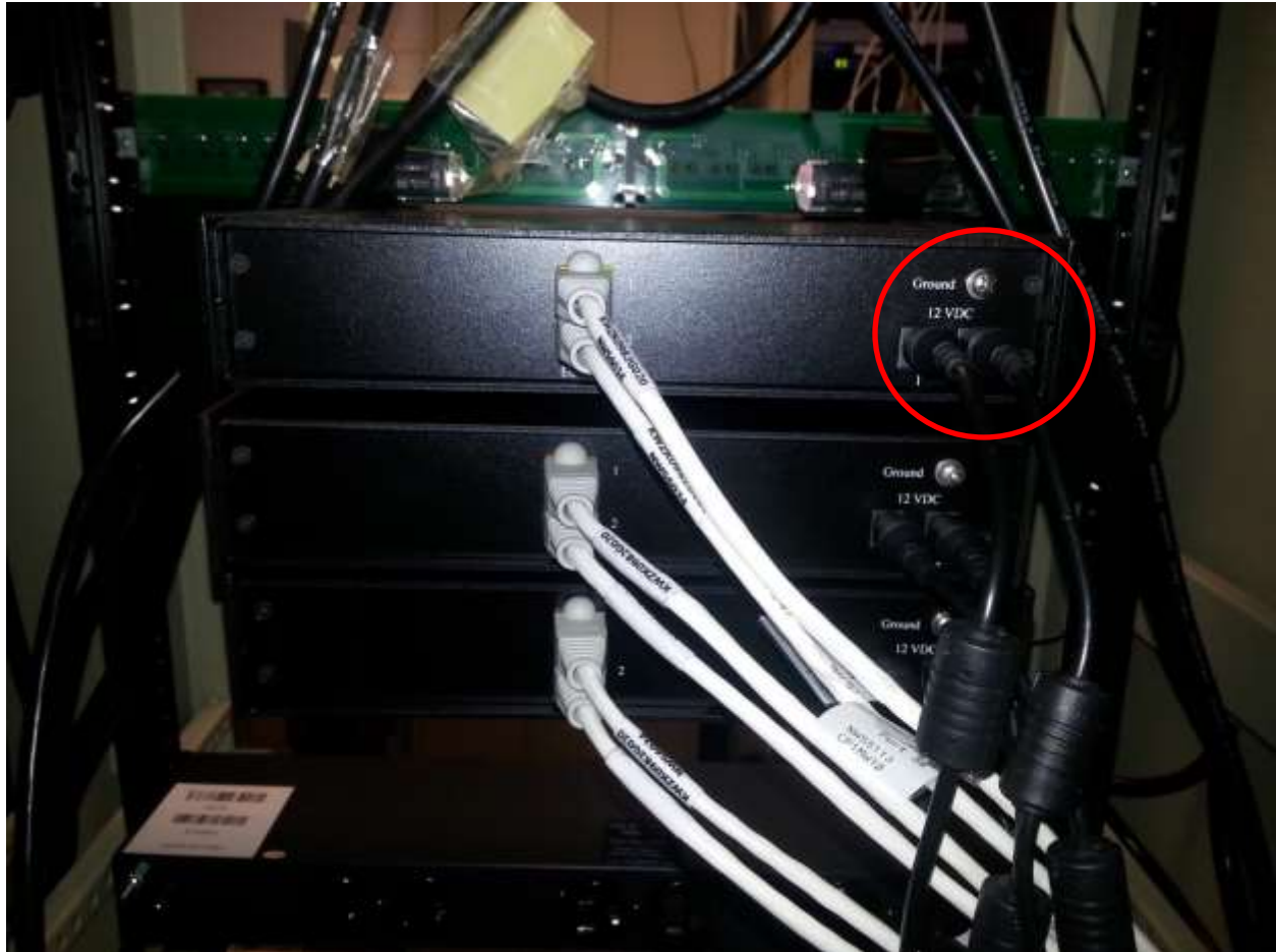
Exhibit 32.6-1 Front view of Rack 1; circle indicates power cables for DAC1
