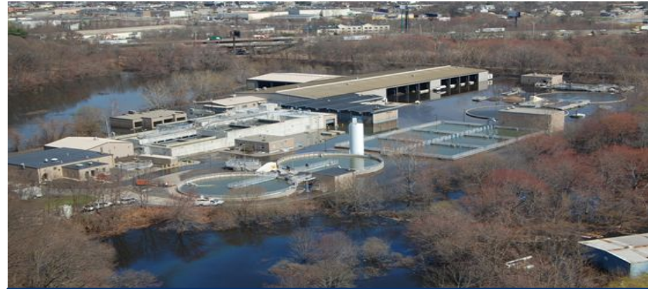
West Warwick Wastewater Treatment Facility under siege, morning of April 1st, 2010 as the Pawtuxet River began to recede. Photo: RI ANG
